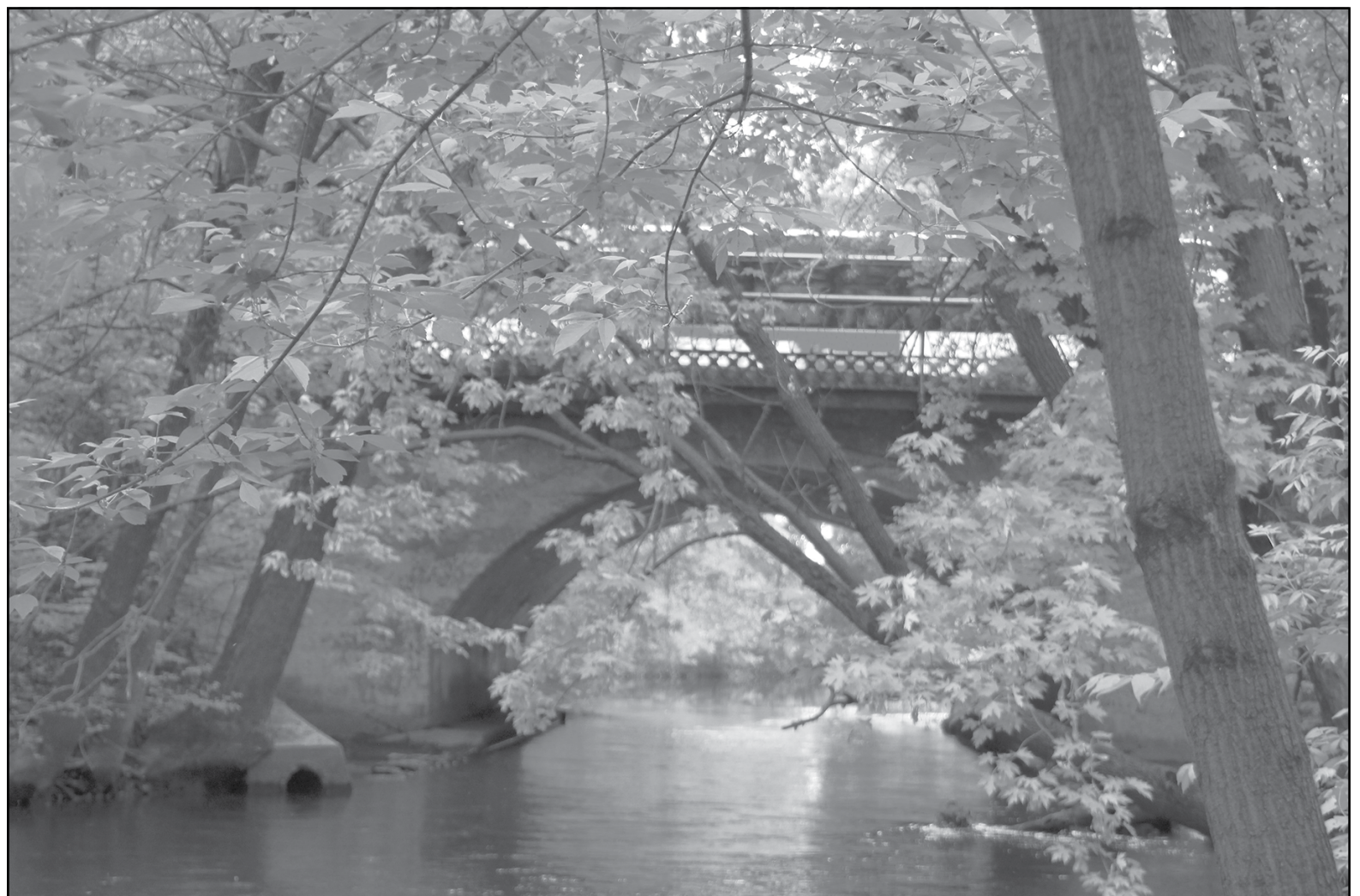
When the new bridge is completed in 2019, trail users will cross under the busy S. 28th Ave. roadway along Minnehaha Creek. (Photo by Tesha M. Christensen)
