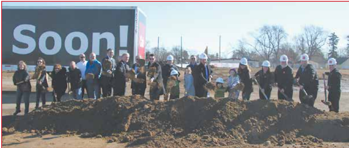
Representatives from Cub, development staff members, local politicians, and neighborhood children break ground for the new CUB store at 46th and Hiawatha, just east of the Holiday station store on Thur., Mar. 15. The new urban-style grocery store is expected to open in one year.
