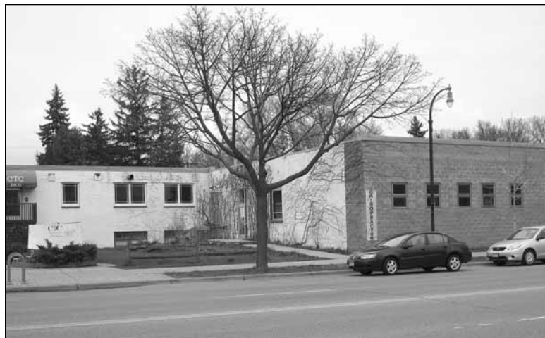
Remodeling projects often surprise a new owner, and the building at 3400 E. Lake St. was no exception. "There was asbestos and lead paint in both buildings," owner Dan Kennedy noted. (Photo by Jan Willms)
