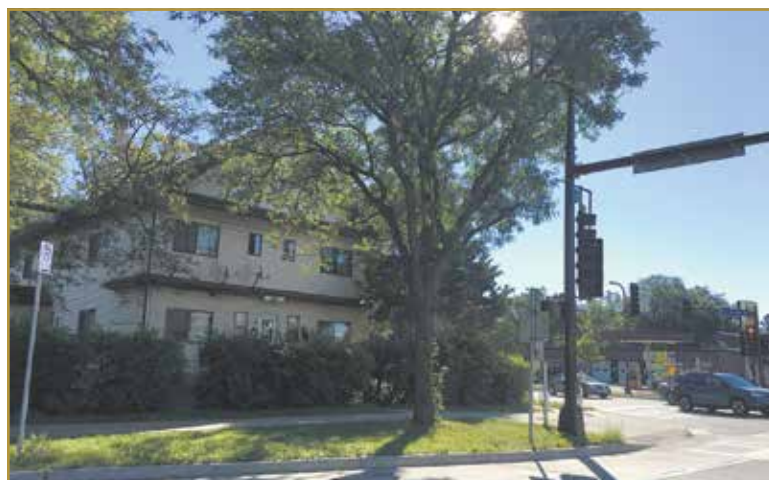
The existing building at the corner of 46th St. and Minnehaha Ave. offers 12 transitional housing units that share four bathrooms with low-cost rents ranging from $450-650 a month. Sweeney said they considered keeping the building, but determined it was too run-down to rehabilitate. It will be replaced with a five-story structure that will have 54 apartments and retail space on the first floor. (Photo by Tesha M. Christensen)
