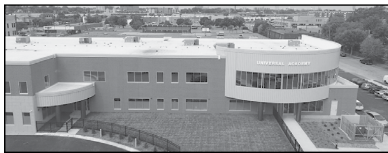
Universal Academy Charter School moved into a 19,600-square-foot second-story addition built on the back side of the building in time for classes to begin for the 2018-19 school year. (Photo submitted)
