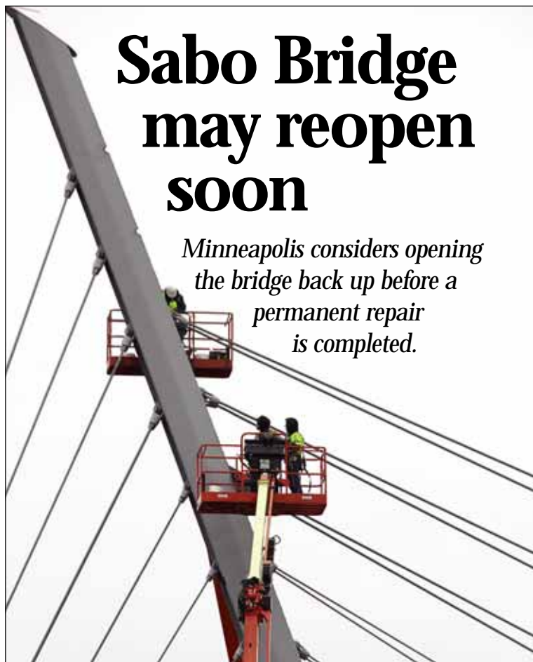
Workers install a variety of equipment on the Sabo Bridge in order to collect data about how the bridge responds to weather conditions. That data will be used to help fashion a repair plan. (Photo by Tesha M. Christensen)
