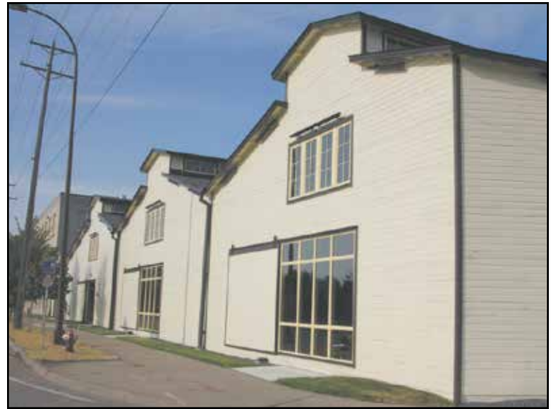
Once home to Lake Street Sash and Door Company, this brick building and adjacent shed now offer 78 affordable housing units, courtesy of a project completed by the Plymouth-based Dominion, Inc. The project wrapped up in July 2016, and renters began moving in during August. A month later, 100 percent of the lofts had been rented out. Residents come from within a few miles of the site, drawn in by a banner on the building, flyers at local businesses, handouts at the light rail station at 38th, and word of mouth. (Photo by Tesha M. Christensen)
