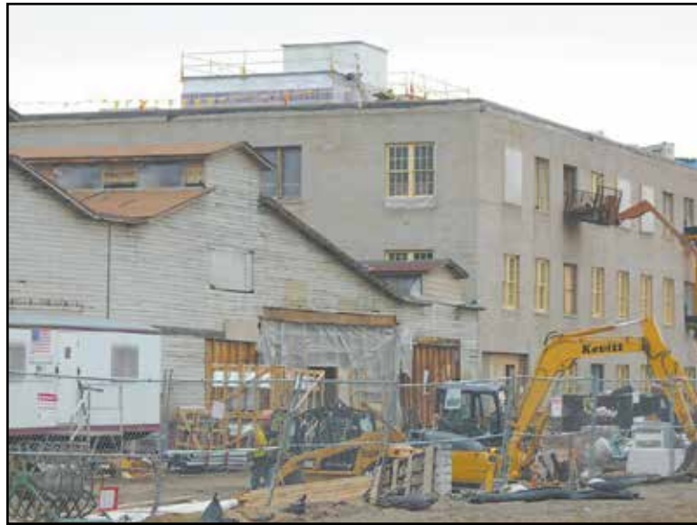
To restore the buildings to their historic look, paint was removed from the bricks on the northern building. On the southern side, metal sheeting was removed to showcase the original clapboard siding. The project was funded in part by historic preservation grants. (Photo submitted)
