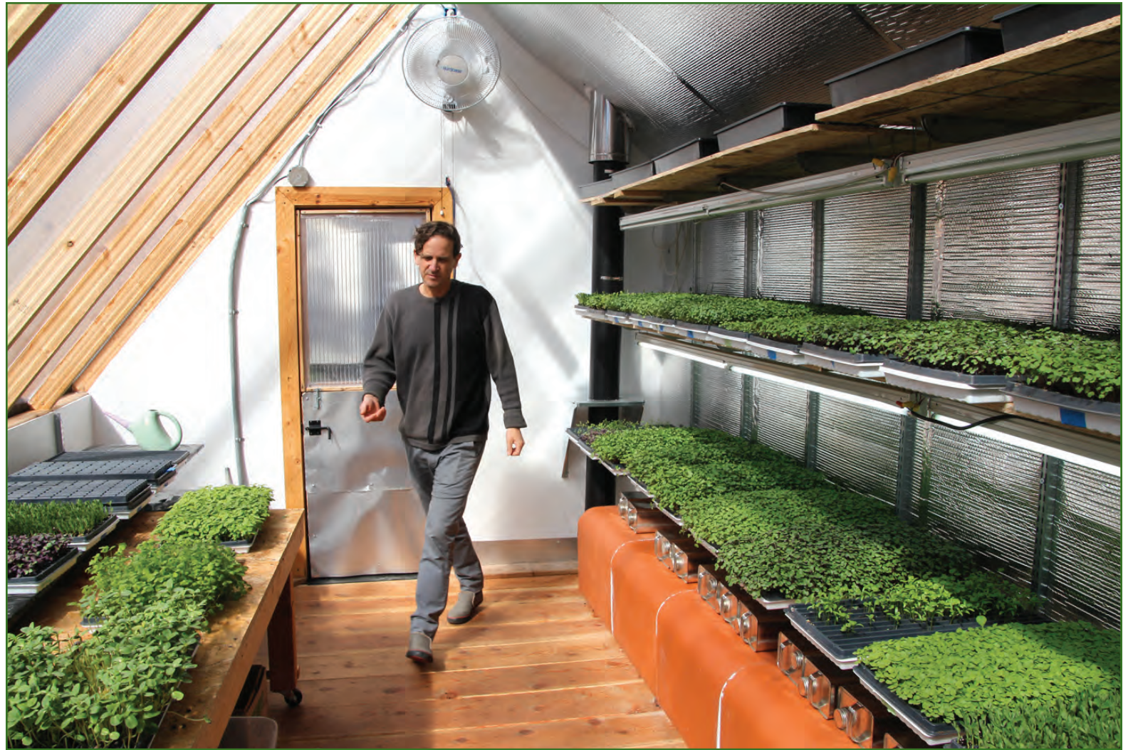
David Thiel explains how his deep winter greenhouse works, using a combination of insulation and water to absorb and retain heat. He intends to begin offering consulting services and plans so that others can build their own deep winter greenhouses to grow food year-round. (Photo by Tesha M. Christensen)
