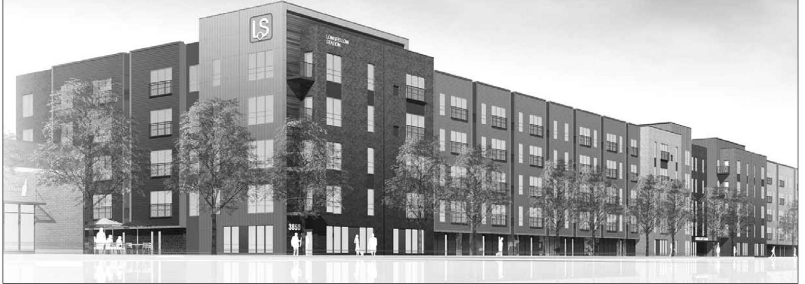
After a series of lengthy delays, work has finally begun on the long-awaited Longfellow Station at the 38th and Hiawatha. The $31 million project will provide a new supply of mixed-income rental housing on the former Purina Mill site. The project will also include a 10,000 square foot commercial building across from the 38th Street LRT station.
