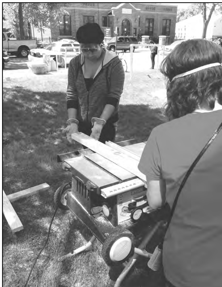
Students are gaining construction experience while also putting math and science skills to real-life situations. (Photo submitted)
