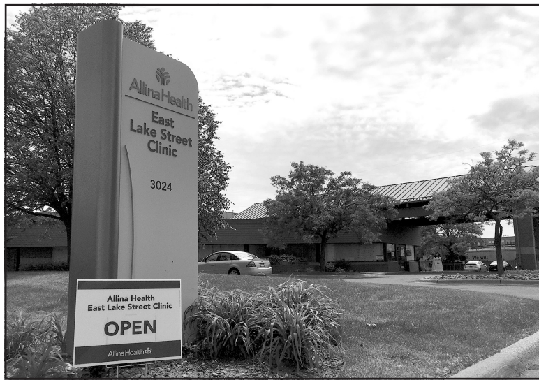
Although the Arby's to the north was burned to the ground and the Third Precinct across the street set on fire, the East Lake Street Clinic was not damaged during the protests. (Photo submitted)
