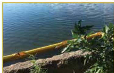
The city of Minneapolis installed a trash curtain to contain the garbage coming out from the storm water sewer directly into the lake in August. (Photo submitted)
