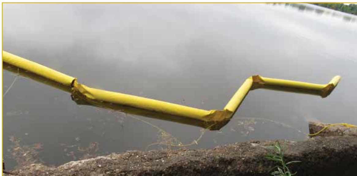
Within a few days of being installed, the trash curtain came unmoored following a heavy rain. (Photo submitted)
