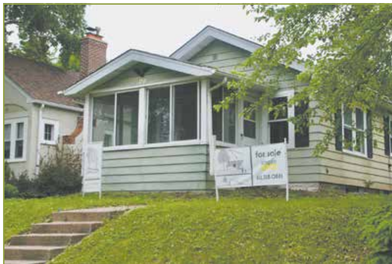
The little house on 13th Ave. is still in the 'before' stage of remodeling. (Photo by Stephanie Fox)
