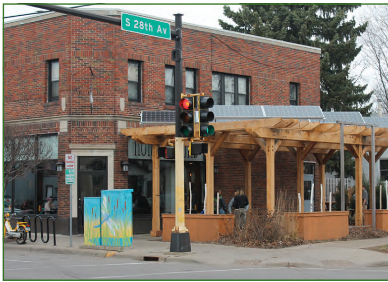
In addition to solar panels on the outdoor patio, Northbound Smokehouse and Brewpub has an array on the roof. In total there are 68 panels, with the ability to generate enough electricity to power 3.3 homes (or 254 light bulbs) for a full year. It also provides some summertime shade to the patio. (Photo by Loren Green)
