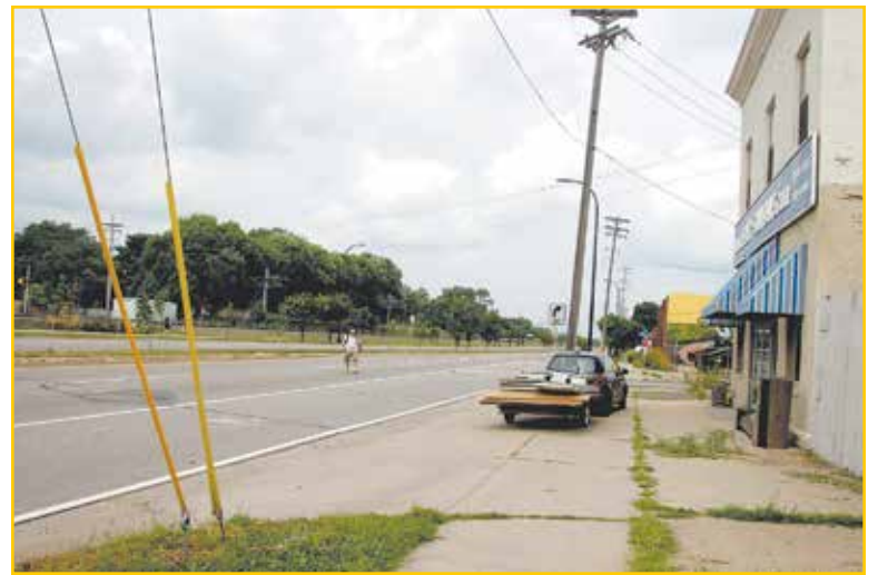
RS Eden President and CEO Dan Cain hopes the city will consider constructing a pedestrian bridge near 45th and Hiawatha to serve residents, including high-density housing projects at Amber Apartments and the Snelling Yards site. Right now, people regularly cross Hiawatha near 45th instead of walking down to the crosswalk at 46th. (Photo by Tesha M. Christensen)
