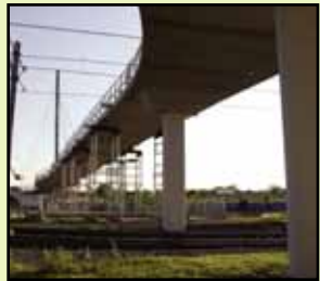
Sabo Bridge reopens June 4
