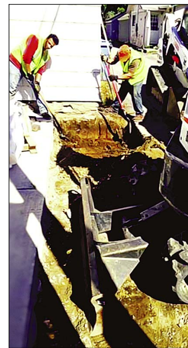
Five properties in the demonstration project installed raingardens, which are bowl-shaped gardens that use deep-rooted plants to hold and soak up stormwater.
