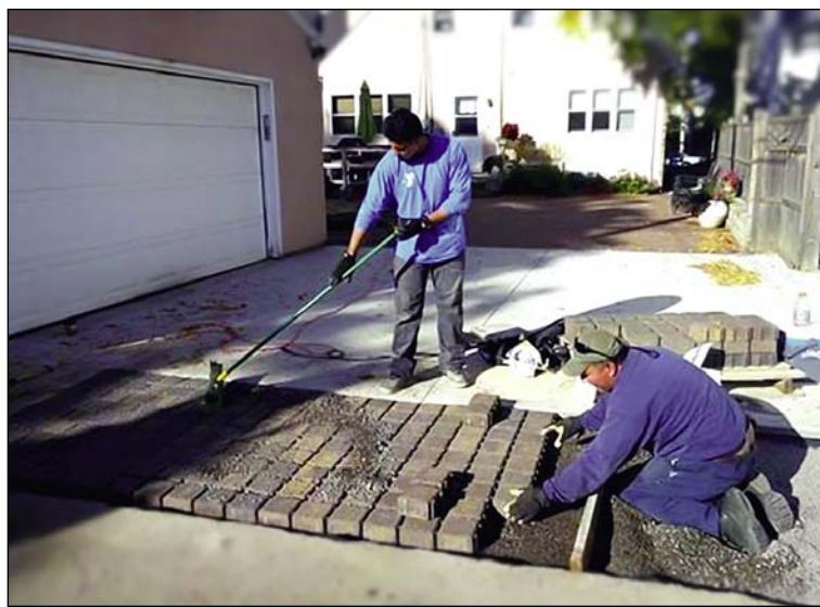
Four properties in the demonstration area installed strips of pavers that allowed rainwater and water runoff to pass through to the soil.
