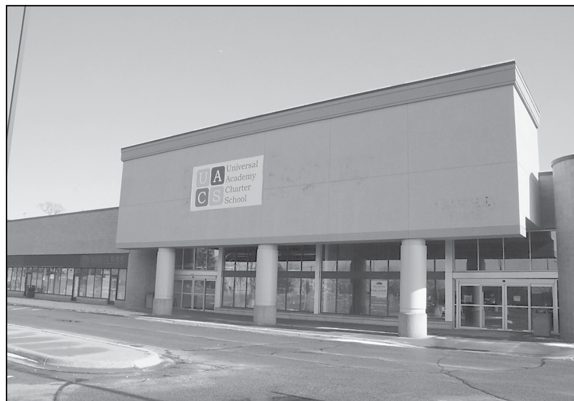
The former Rainbow Foods site has been mostly vacant since the grocery store closed in 2014. It had been purchased by Jerry's Enterprises as part of a 27-store deal that reshaped the Twin Cities grocery scene. The building and 6-acre lot were purchased by Wellington two years later for $5.35 million, according to Hennepin County records. Universal Academy Charter School moved into temporary classrooms in time to start the 2017-18 school year. (Photo by Tessa M. Christensen)
