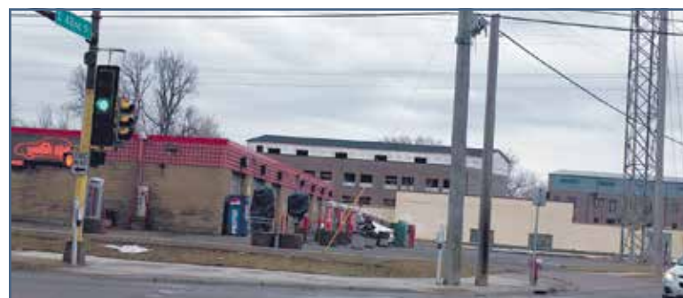
A proposal before the city would tear down the existing Wash Me car wash and replace it with two one-story buildings to house a Starbucks and Domino's Pizza. (Photo by Tesha M. Christensen)
