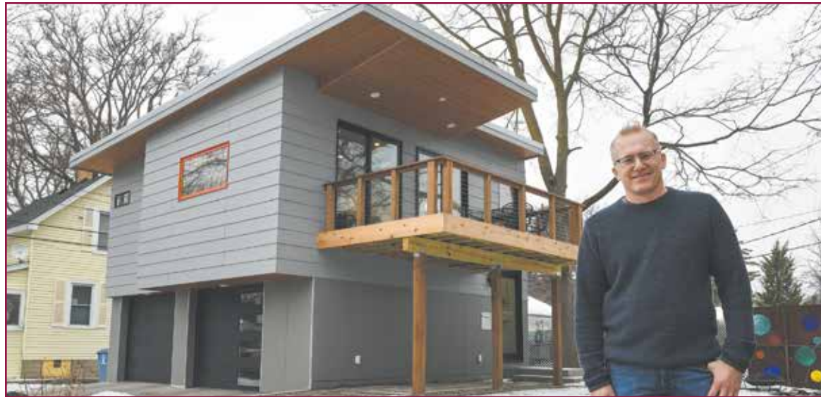
Chris Iverson built his ADU above his garage in the back of his duplex. By law, the owner or a relative of the property owner must live in an ADU. (Photo courtesy of the Minneapolis-Saint Paul Home Tour)
