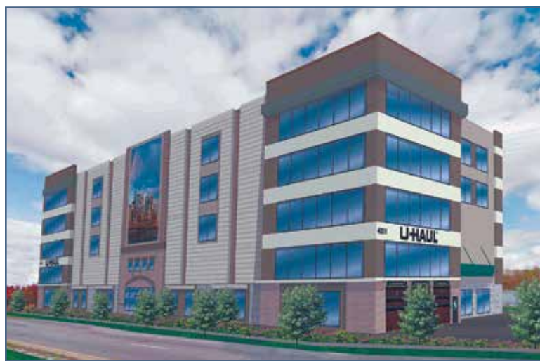
U-Haul plans to raze the large factory building on the south side of the lot to construct a five-story self-service storage center along Hiawatha Ave. south of its intersection with 42nd. The small, historic building on the north side of the lot, formerly housing Taylor Star 1 Automotive, will be turned into a showroom with model storage rooms for rental selection. (Graphic submitted)
