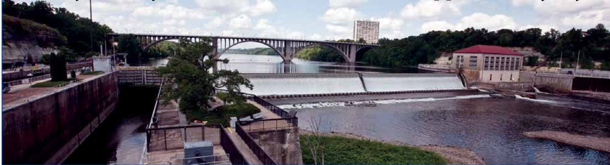
When Lt. Zebulon Pike first explored the Upper Mississippi River Basin in 1805, he described the 8.5 mile stretch of the Gorge as one of continuous rapids. This year marks the 100th anniversary of the Ford Dam (pictured here), one of two dams within the Gorge that have greatly altered the way the river flows. (Photo by Margie O'Loughlin)
