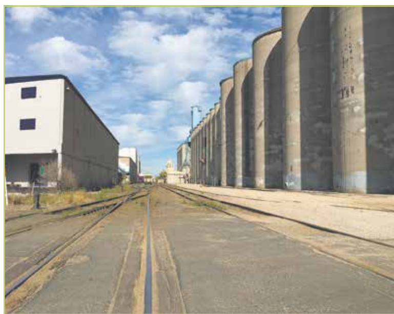
The General Mills grain elevators at 3716 Dight Ave. have been identified as a pilot of the Min Hi Line. The site was recently sold to Hayes Harlow Development, who is also working on a development at 46th St. and Minnehaha Ave. (Photo submitted by the Min Hi Line Coalition)
