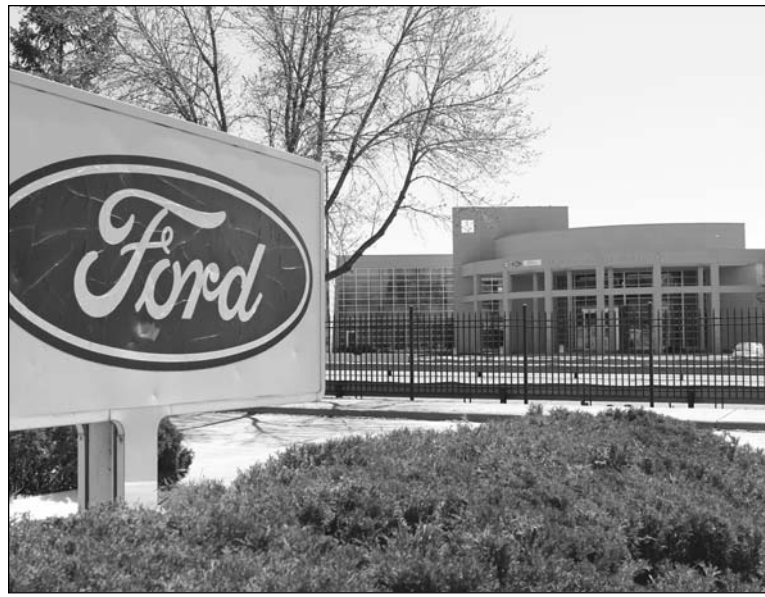
The former Ford Motor Company plant in St. Paul's Highland Park neighborhood will be coming down soon as city and Ford officials work on demolition plans. The plant has been closed for more than a year.
