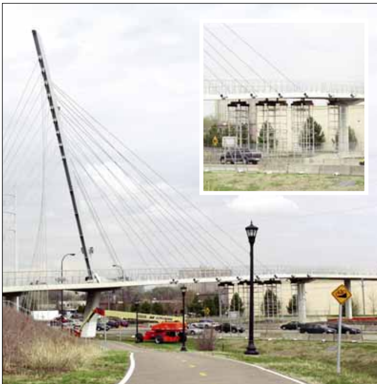
At 10:06 p.m. Feb. 19, a citizen reported finding a pair of cables lying on the Sabo Bridge deck. City workers responded, and discovered that a partly rusted diaphragm plate had fallen 100 feet from the mast, and released the topmost cable, number nine.
