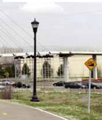
At 10:06 p.m. Feb. 19, a citizen reported finding a pair of cables lying on the Sabo Bridge deck. City workers responded, and discovered that a partly rusted diaphragm plate had fallen 100 feet from the mast, and released the topmost cable, number nine.
