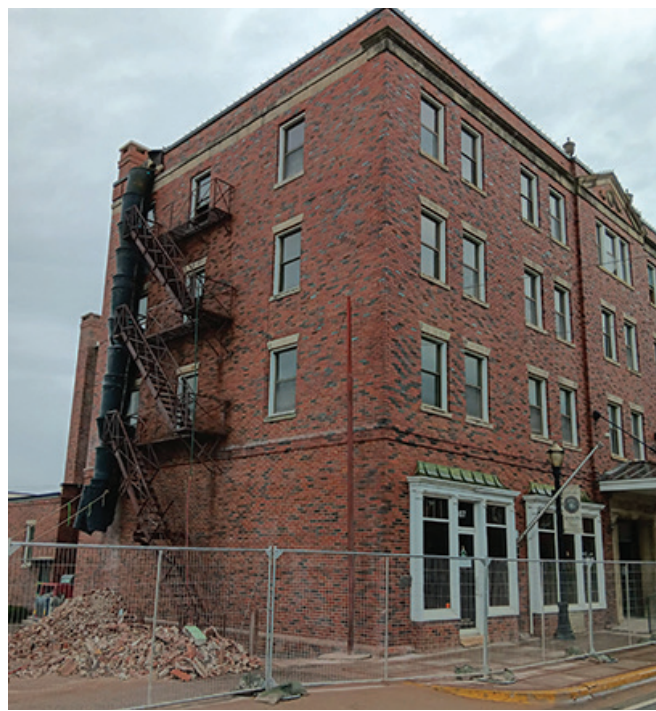
JOHN C COLEMAN BUILDING BEING RENOVATED
