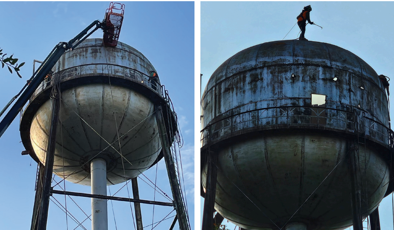
WORKERS PREPARE TO REMOVE OLD WATER TOWER
