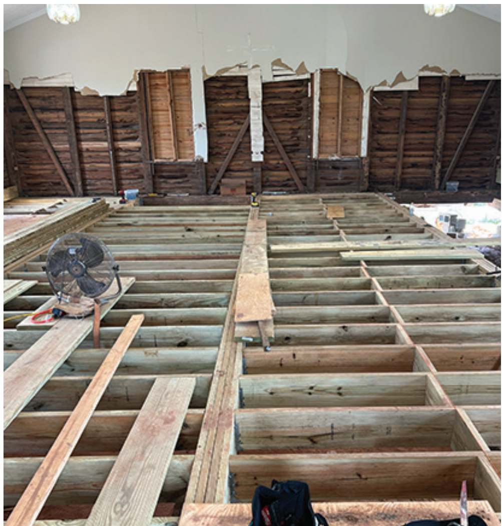
CHURCH BEING RENOVATED
