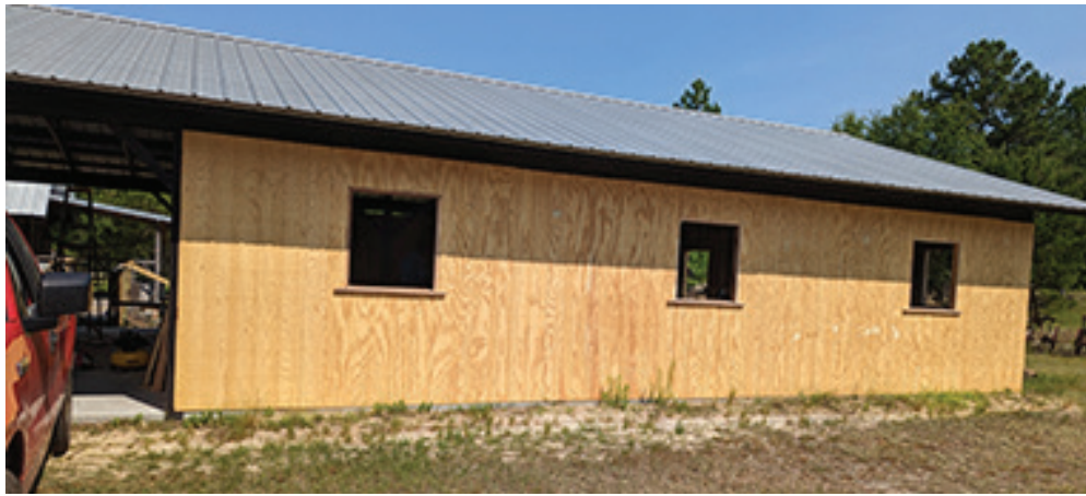
ENCLOSED GROUP SHELTER
