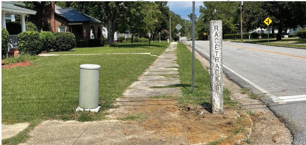
PHOTO OF THE RACETRACK STREET HISTORICAL MARKER THAT WAS REPAIRED
