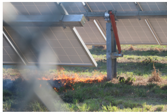
SCENE FROM TWIN CITY SOLAR FARM FIRE Fire at Twin City Solar Farm
