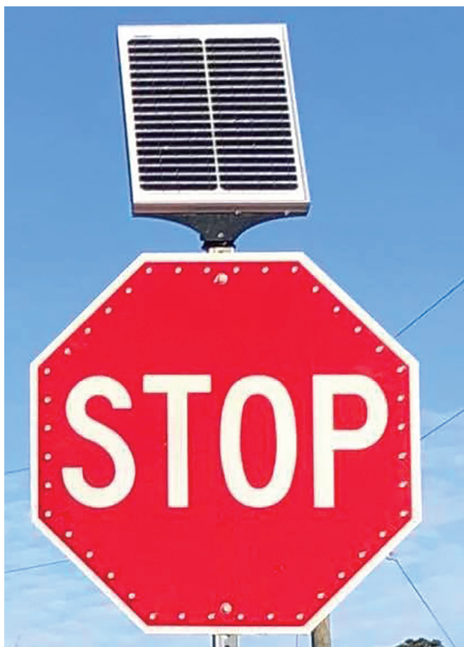
STOP SIGN AND SOLAR-POWERED LIGHT
