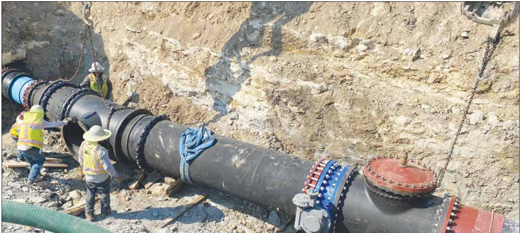
The final connection of the water line from Fort Worth to Willow Park is in place. The red and blue bands are where the two segments were joined. The section with the red circular structure at the top is the valve.
